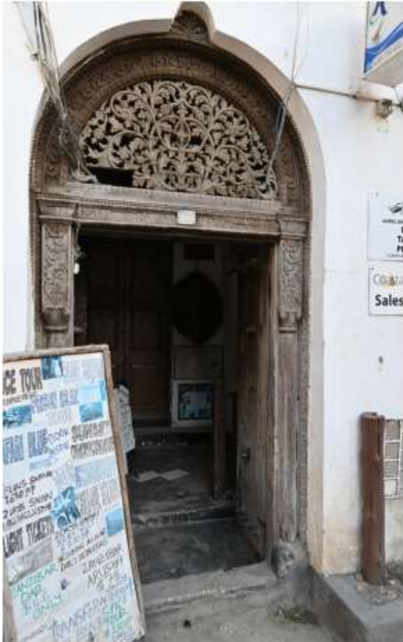
Figure 11: The Indian-style Zanzibar door features an openwork grating and floral designs on a semicircular lintel (Jasiński, 2021)
